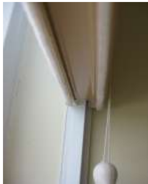
double brush weatherstrip on bottom edge of shade, one similar WS on top edge
